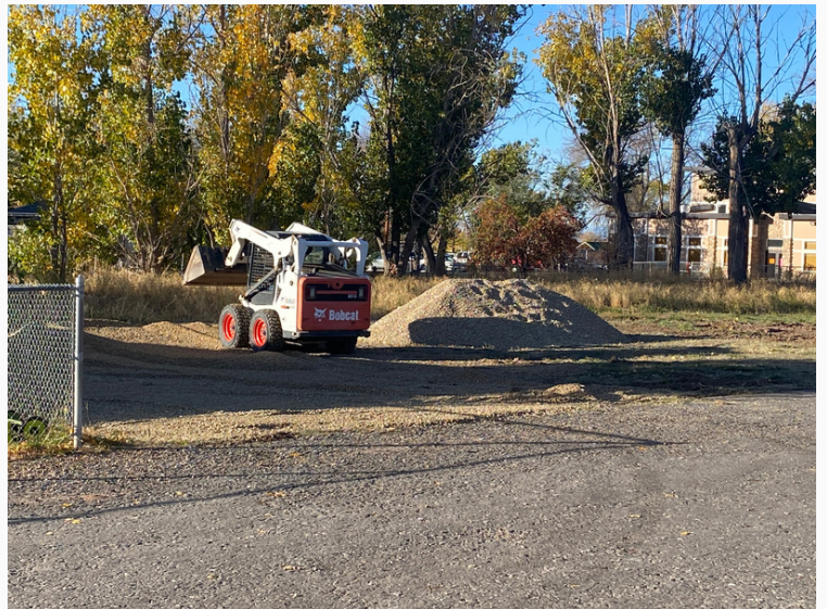
Spreading gravel on our parking area
